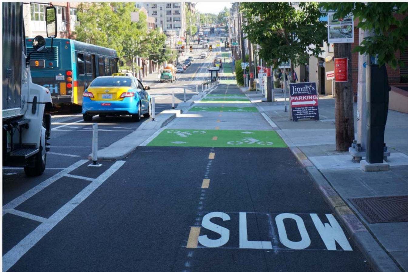
Driveway crossings on Broadway Cycle Track, First Hill Streetcar, Seattle, WA
