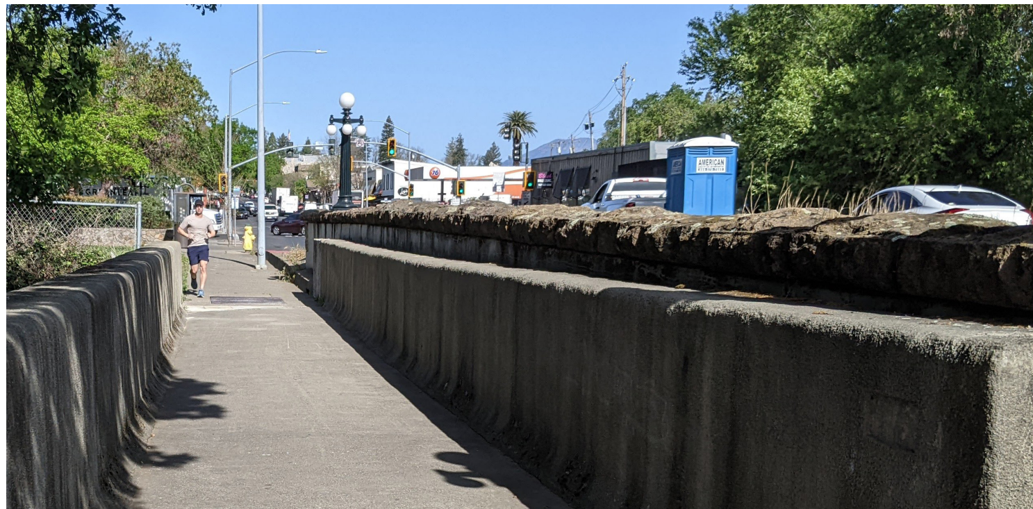
Existing Sulphur Creek Bridge
