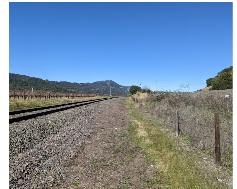
East side of tracks near Station A40+00 (looking north)
