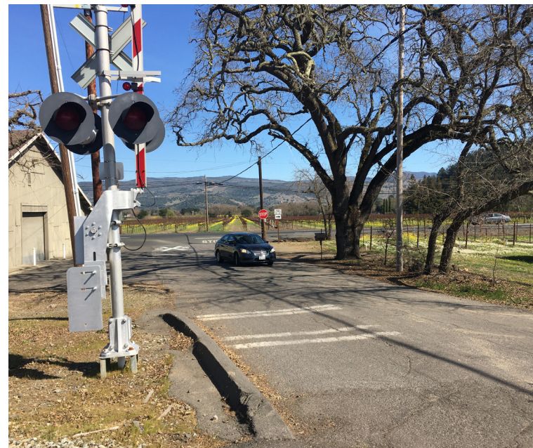
Controlled crossing at Dwyer Road
