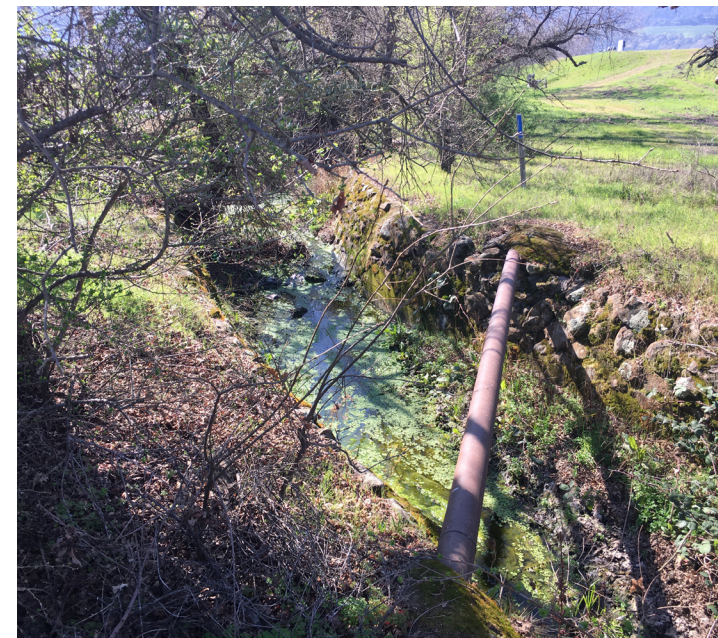
Waterway to be crossed near pump station
