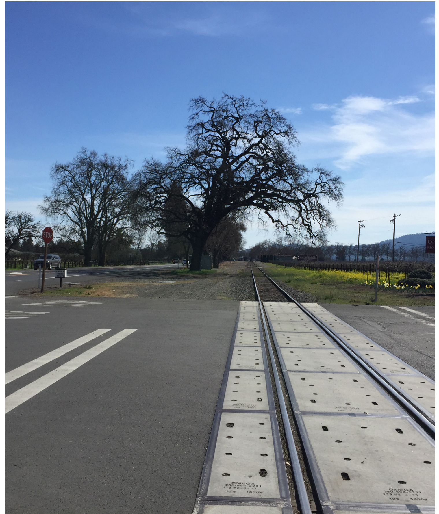
Example of uncontrolled rail crossing
