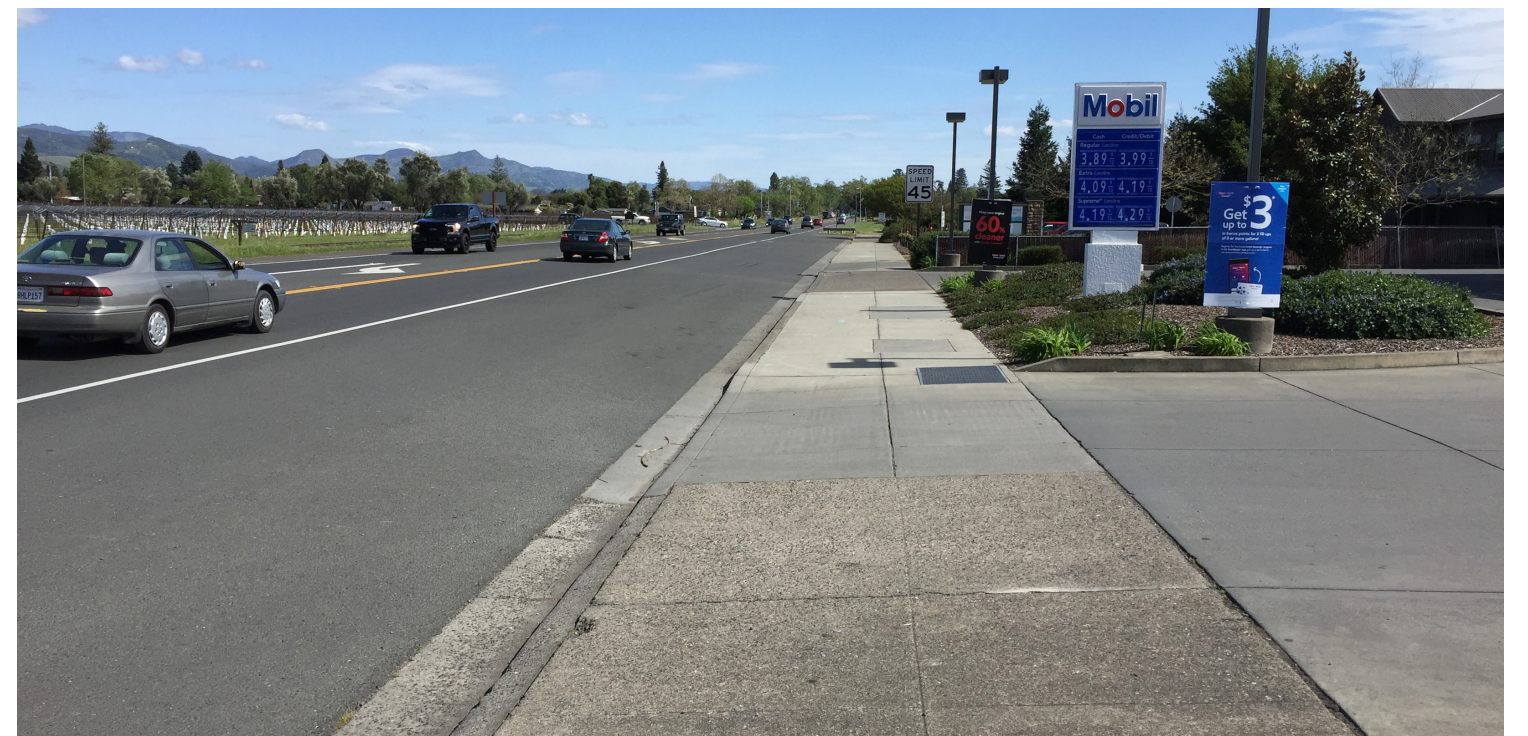
The wide sidewalk south of Inglewood could be adapted for trail use.
