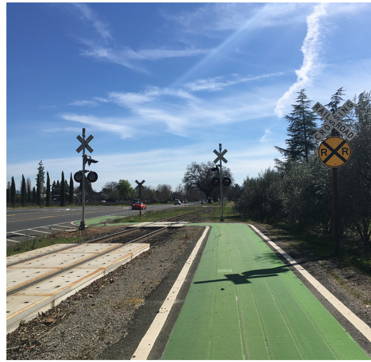
Existing green bike lane
